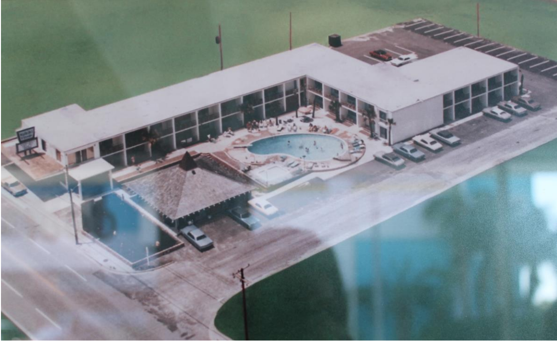
Figure B.1 Waikiki Village after 1967-1969 addition. (Photo courtesy of Nancy Watts Hall.)
