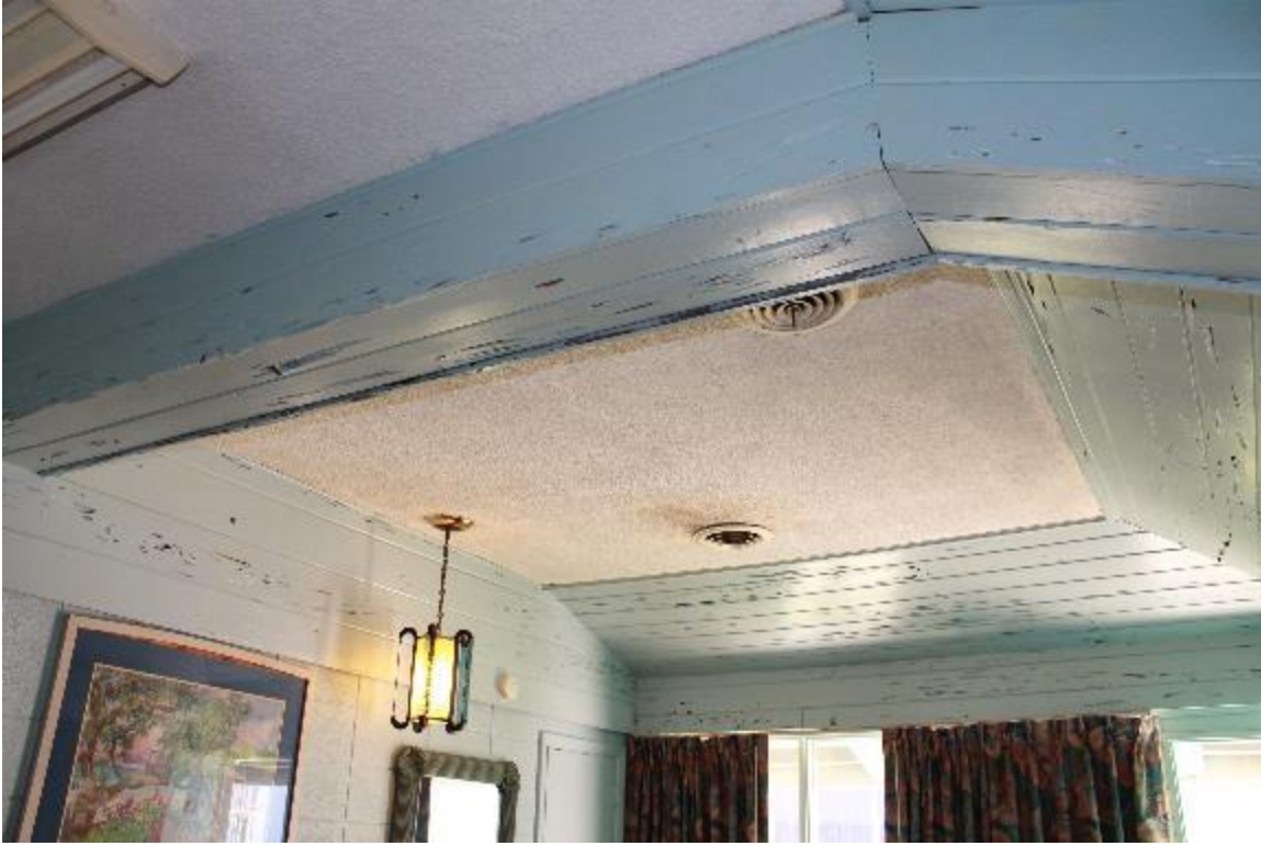
Figure 2.22 Pecky Cypress ceiling framing in Hawaiian-style hut. (Photo by the author.)
