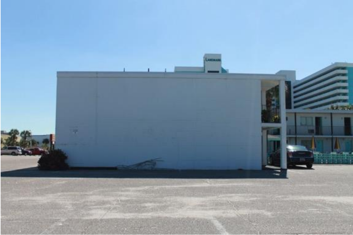
Figure 2.7 West elevation, 1967-1969 addition. (Photo by the author.)
